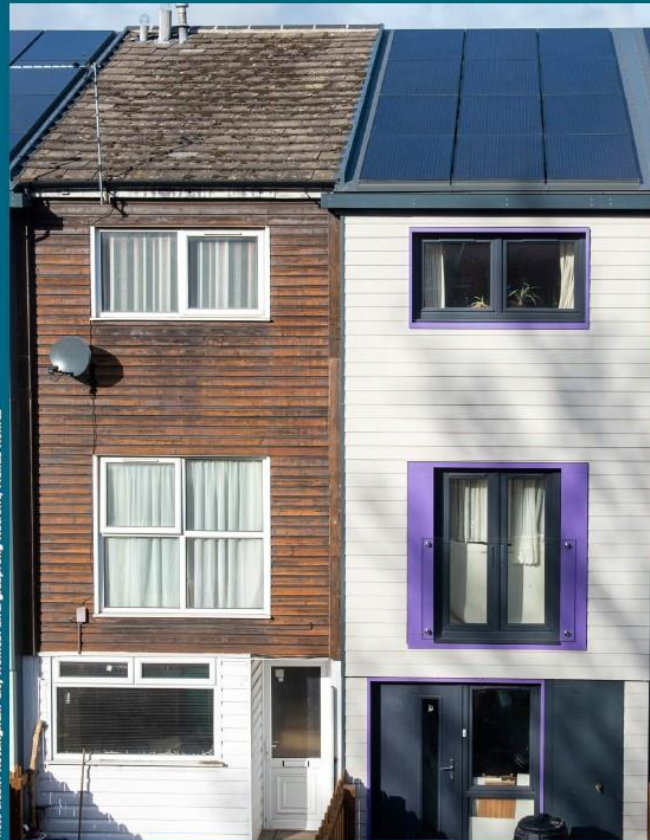
Photo credit: Nottingham City Homes: Energysprung Retrofit, Mellus Homes
