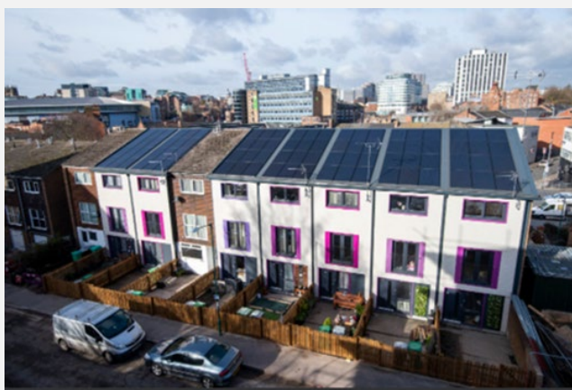
Energiesprong retrofits in Nottingham
